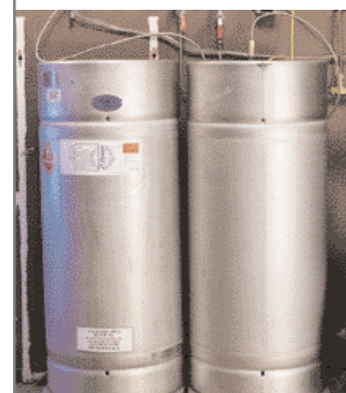
Pipes are installed to run from the containers to each laboratory. One container can feed several laboratories.
